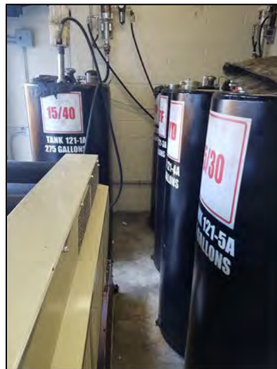
275-Gallon Tanks for Motor Oil, Automatic Transmission Fluid, and Hydraulic Oil (121-VM-1A through 121-VM-5A) Inside Room 121-1 of Vehicle Maintenance Shop (Building 121)
