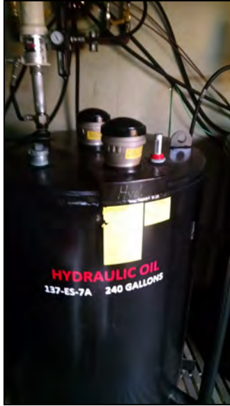
240-Gallon Tanks for Motor Oil, Automatic Transmission Fluid, and Hydraulic Oil (137-ES-6A through 137-ES-8A) Inside Shed behind Heavy Equipment Shop (Building 137)
