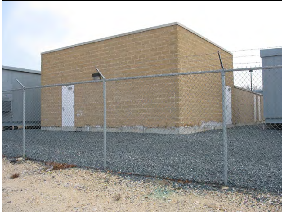
Transformers at North Substation (NS-1T, NS-2T, NS-3T)
