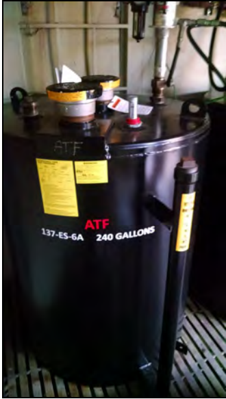
240-Gallon Tanks for Motor Oil, Automatic Transmission Fluid, and Hydraulic Oil (137-ES-6A through 137-ES-8A) Inside Shed behind Heavy Equipment Shop (Building 137)
