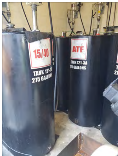
275-Gallon Tanks for Motor Oil, Automatic Transmission Fluid, and Hydraulic Oil (121-VM-1A through 121-VM-5A) Inside Room 121-1 of Vehicle Maintenance Shop (Building 121)
