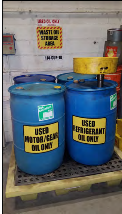
Drum Storage Area (114-CUP-1D) at Central Utility Plant - Building 114
