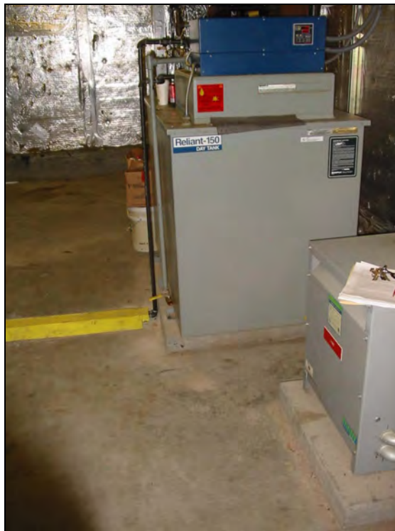
150-Gallon Diesel Fuel Emergency Generator Day Tank (E-3A) On Roof of Pier E (International Terminal)
