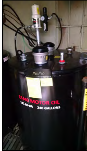
240-Gallon Tanks for Motor Oil, Automatic Transmission Fluid, and Hydraulic Oil (137-ES-6A through 137-ES-8A) Inside Shed behind Heavy Equipment Shop (Building 137)
